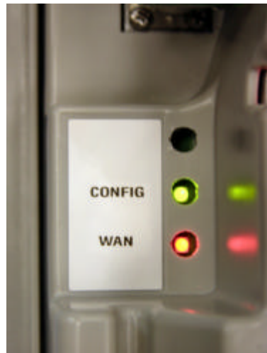
Figure 4 The green programming CONFIG LED indicating communication to the LAN Controller.
