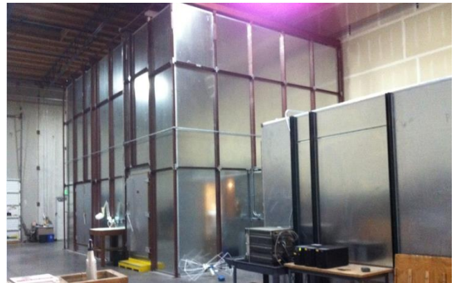
Chamber 2- 3m Semi-Anechoic Chamber (SAC) in Burnaby, BC
