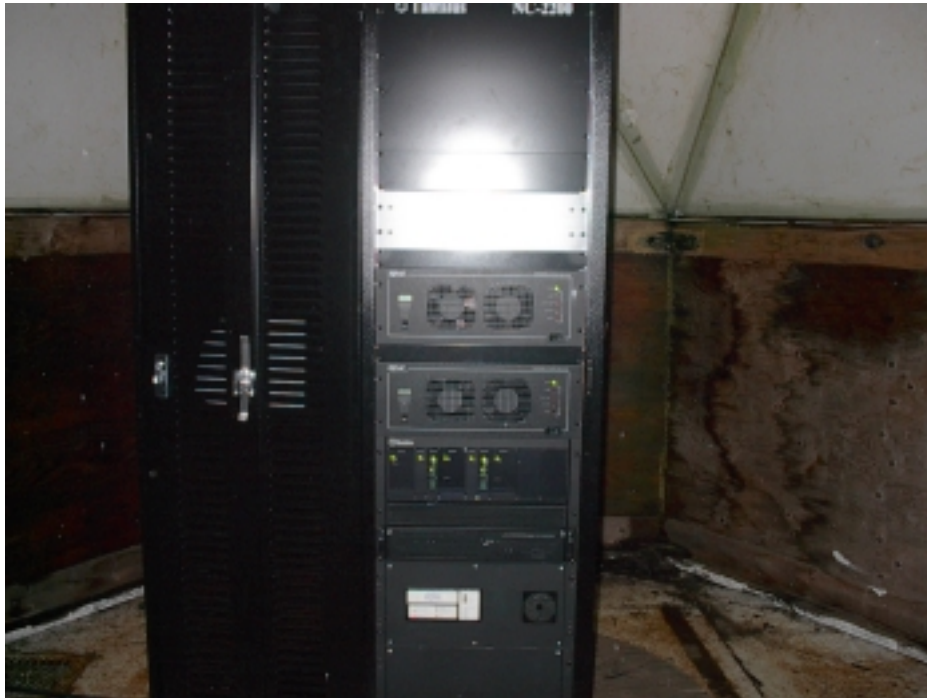
Emissions Test Setup Front View
