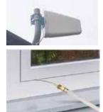
The connector of the cable connection part must be glued with black waterproof tape to prevent long-term signal drop and reduce signal loss!
