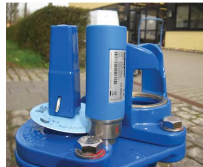
Logger on an underground hydrant
