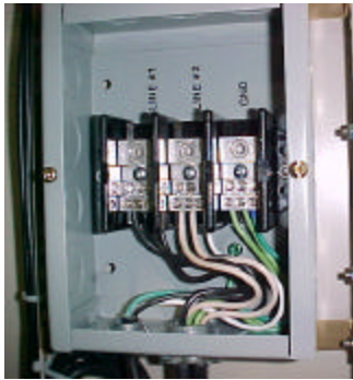
Figure 3-3: AC Input Box Assembly
