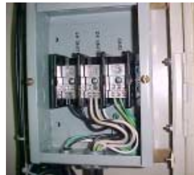
Figure 3-4. AC Input Box Assembly.
