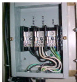
Figure 3-4: AC Input Box Assembly
