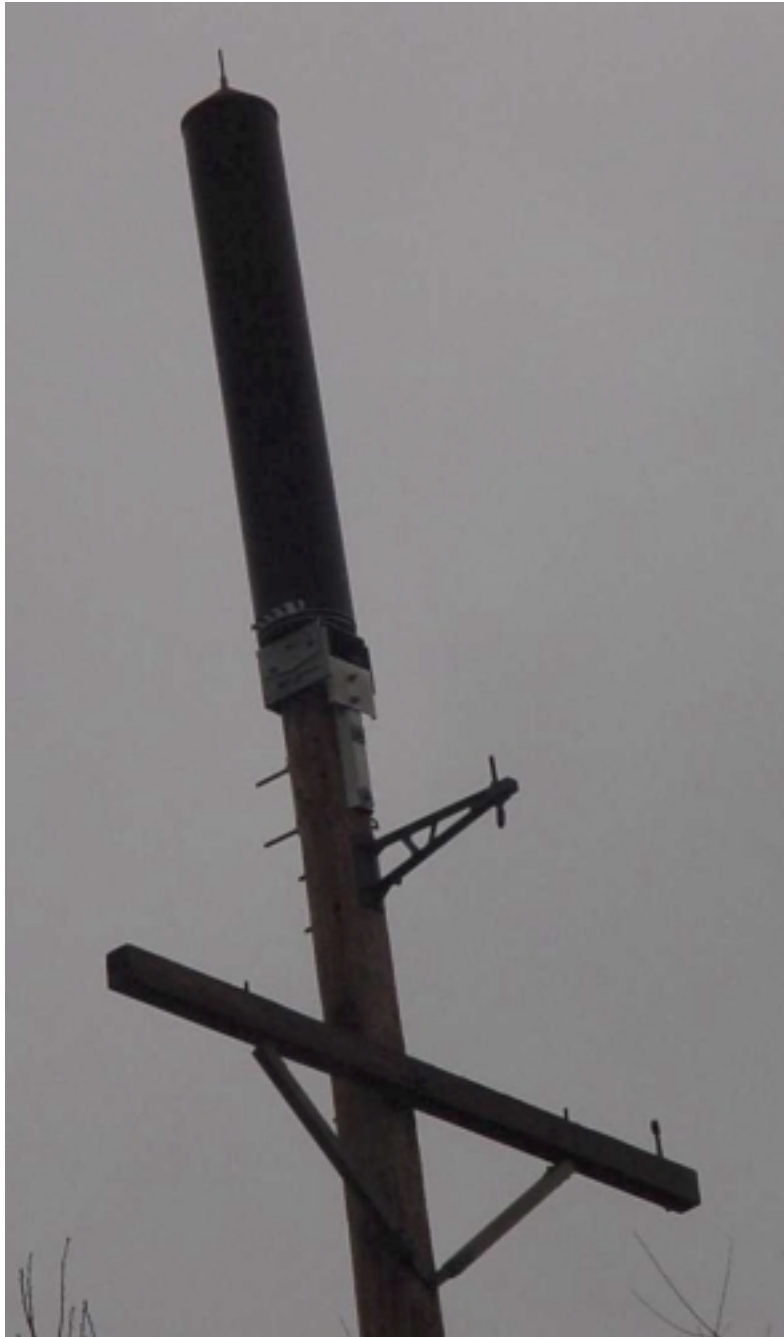
Figure 6-6 RAN Antenna Mounted on Pole
