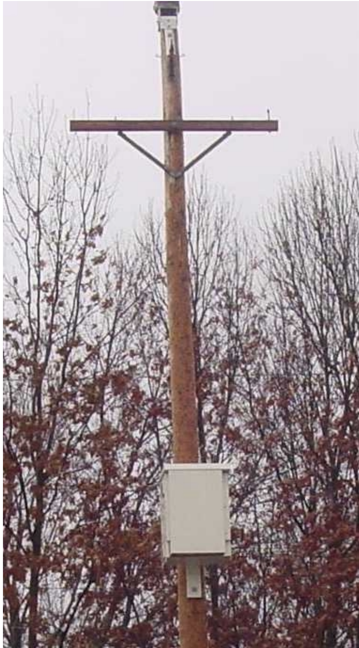
Figure 6-7 RAN Enclosure Mounted on Pole
