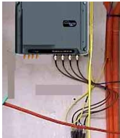
Figure 3-9. Antenna Connections
