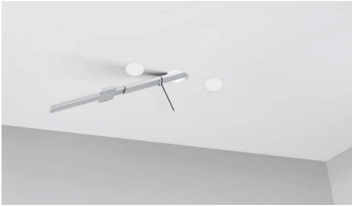
Figure 64. Placing the Bracket I & VI
