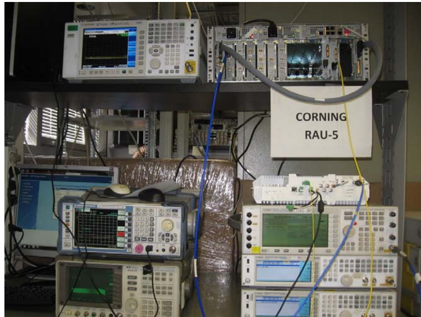
Figure 3. Conducted Emission From Antenna Port Test
