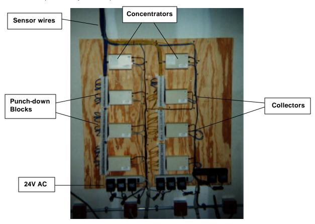
The punch-down blocks, collectors, and concentrators should be installed in a secure location, such as a communication or server room. The installation should allow for wiring access, neat wire routing and dress, and connection of any sensor wire -pair to any collector input. Neat and orderly punch-down blocks are easier to troubleshoot and maintain.
