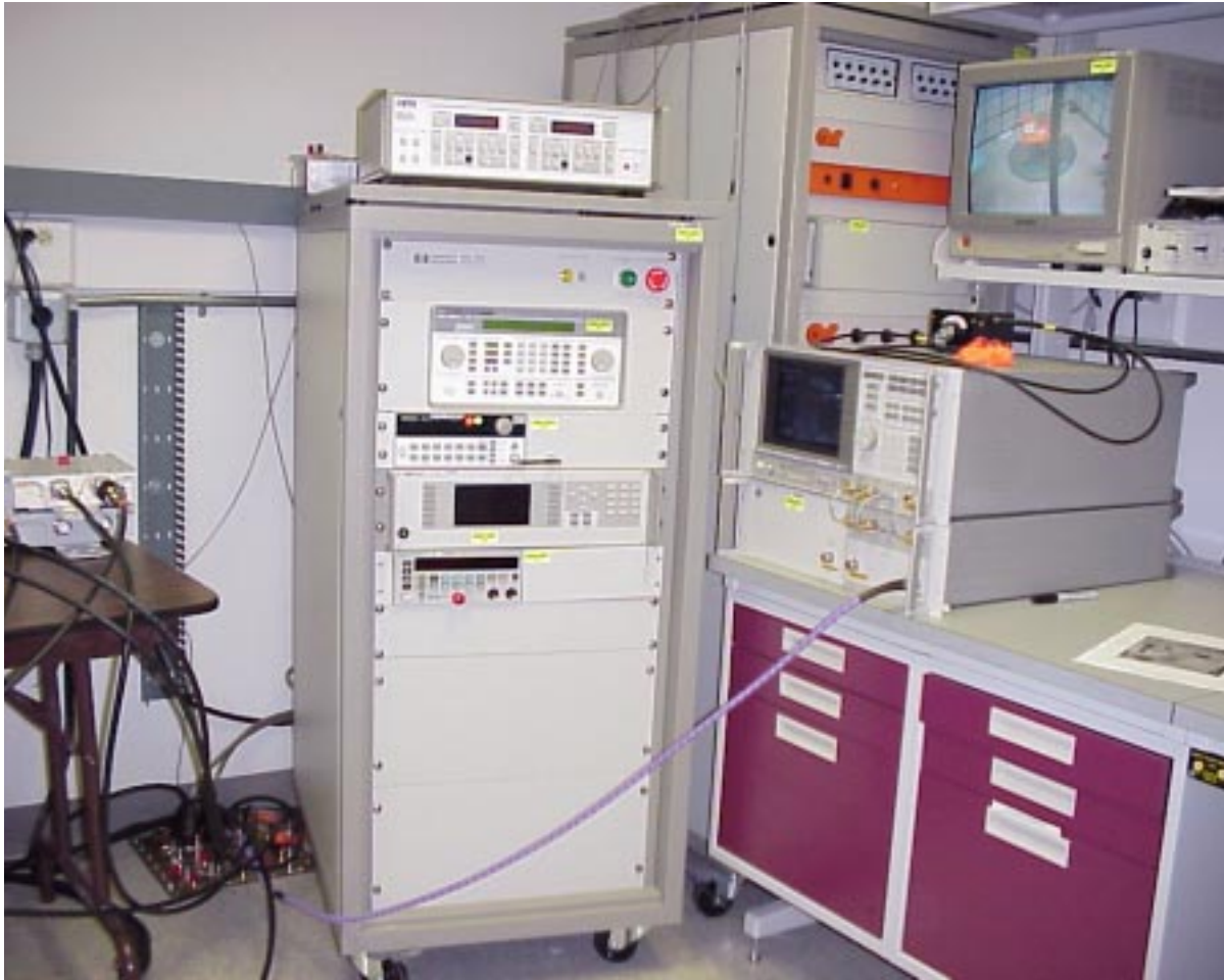
Figure 12.7 3 meter shield room control room
