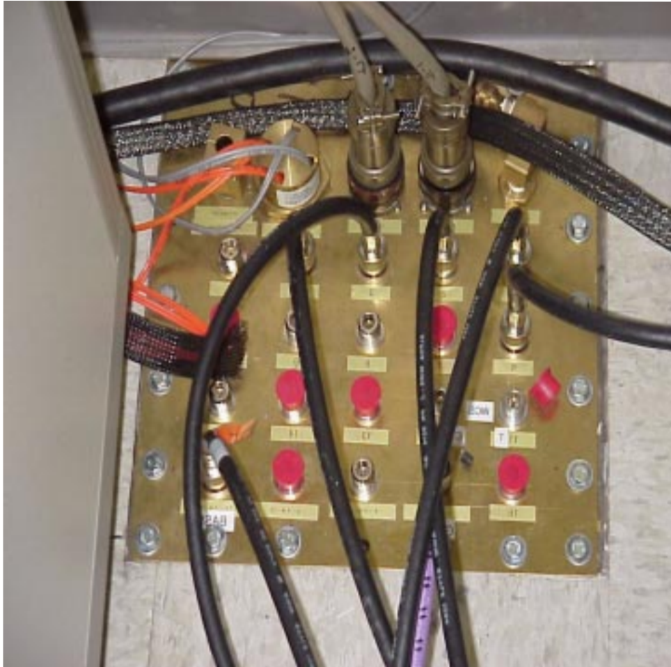
Figure 12.8 3-meter Control Chamber Access Panel Penetration
