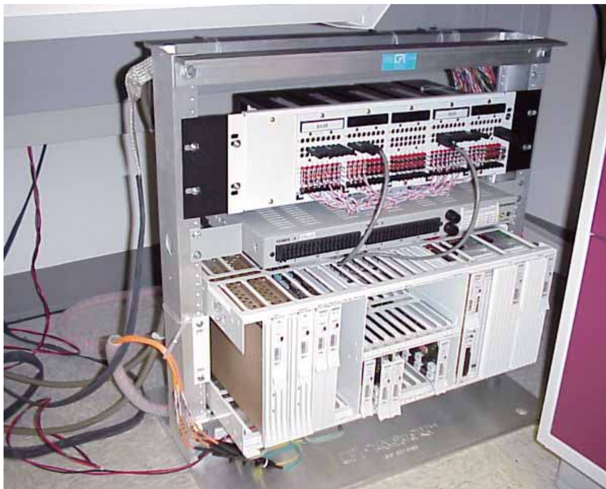
Figure 12.9—T1 fiber optic lines
