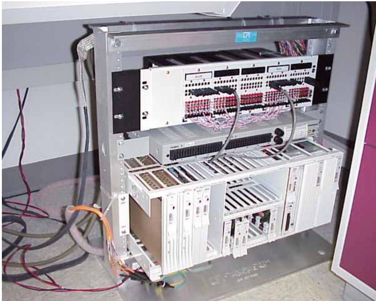
Figure 12.9—T1 fiber optic lines
