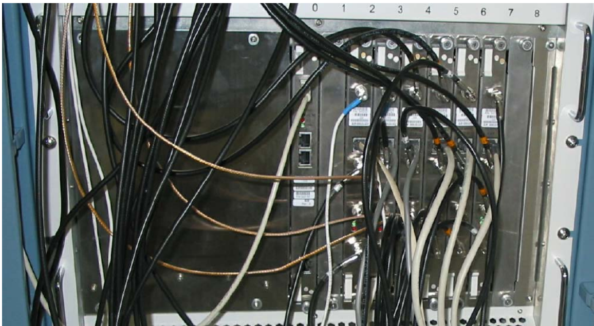
Radio Board 850TRX-Card in Base Station UltraWAVE BTS, AUAC85
