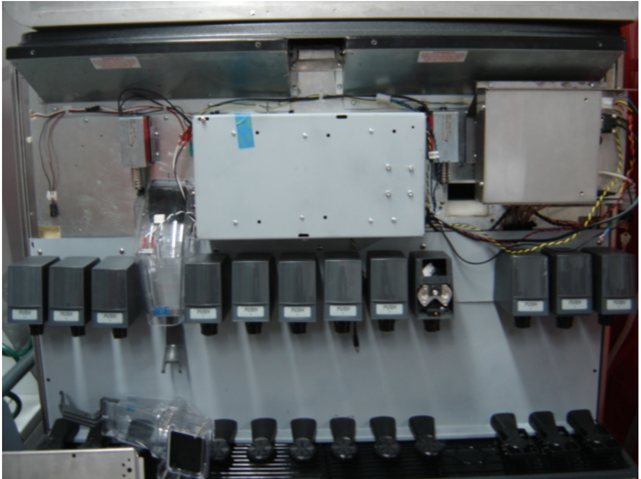
Figure 13: HD011SA003 – Internal View 1
