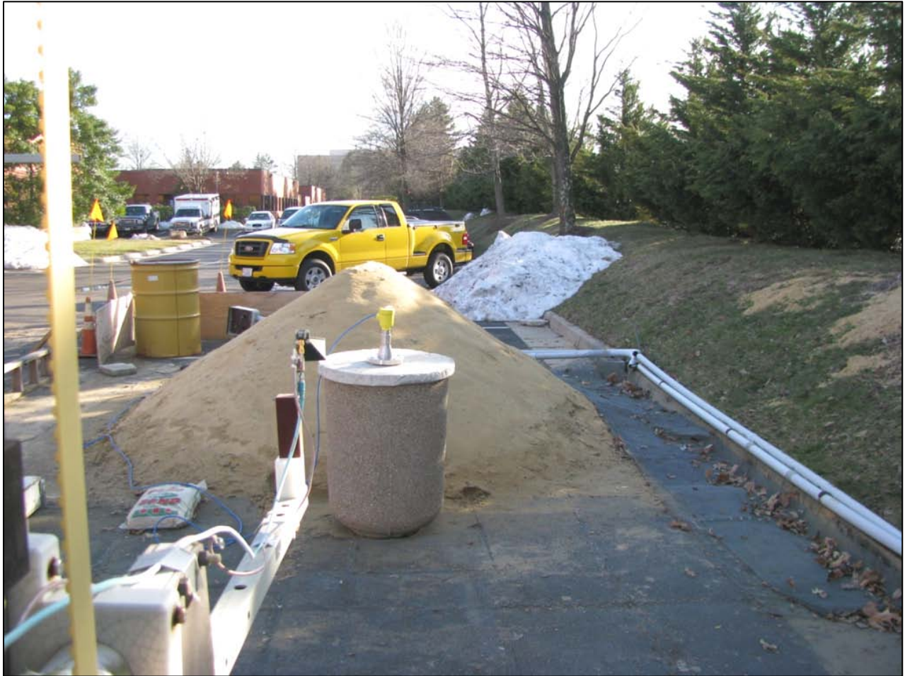
Photograph 25: 75mm Metal Antenna Front View Concrete Tank
