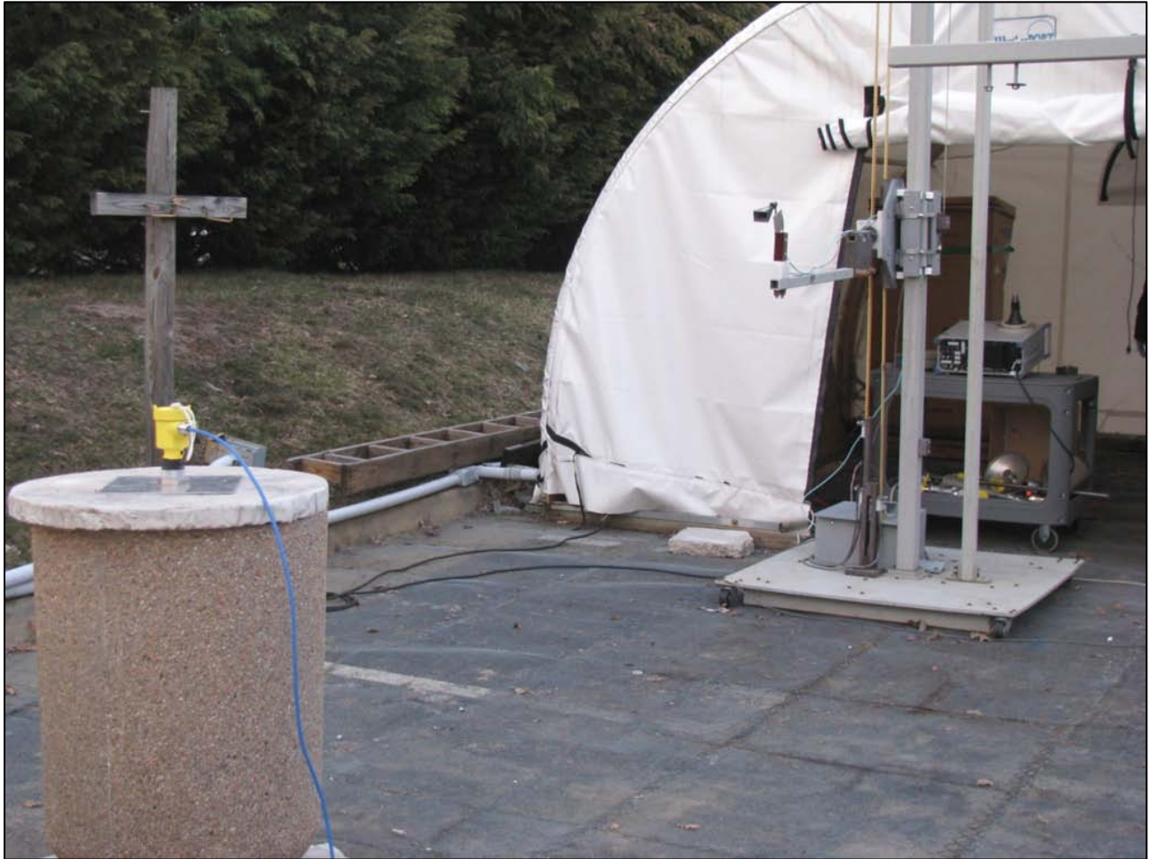
Photograph 32: 1/2" Stub Antenna Rear View Concrete Tank
