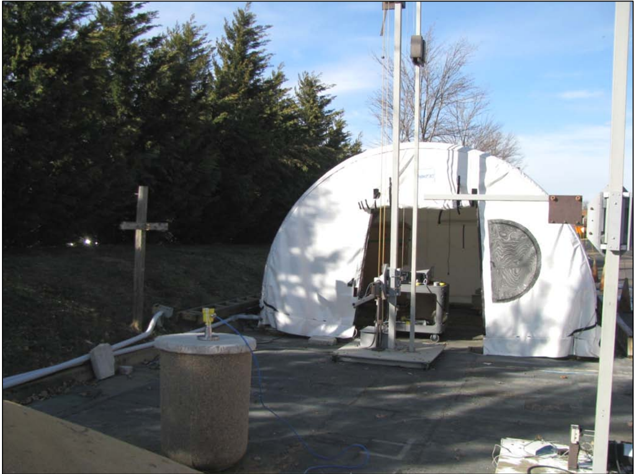
Photograph 28: 48mm Metal Antenna Rear View Concrete Tank
