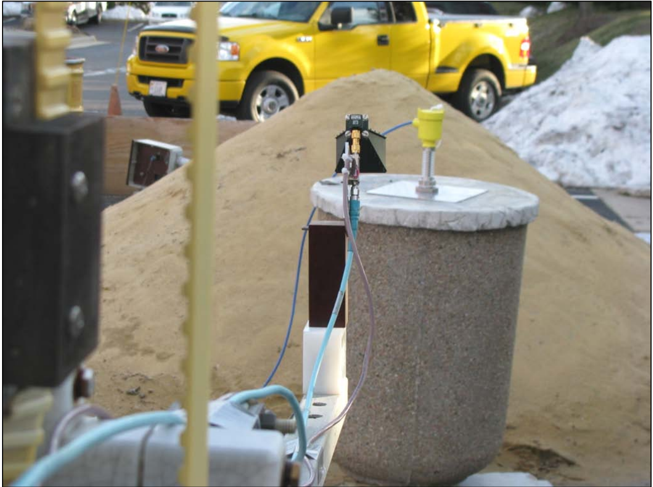
Photograph 20: 245mm Antenna Rear View Concrete Tank
