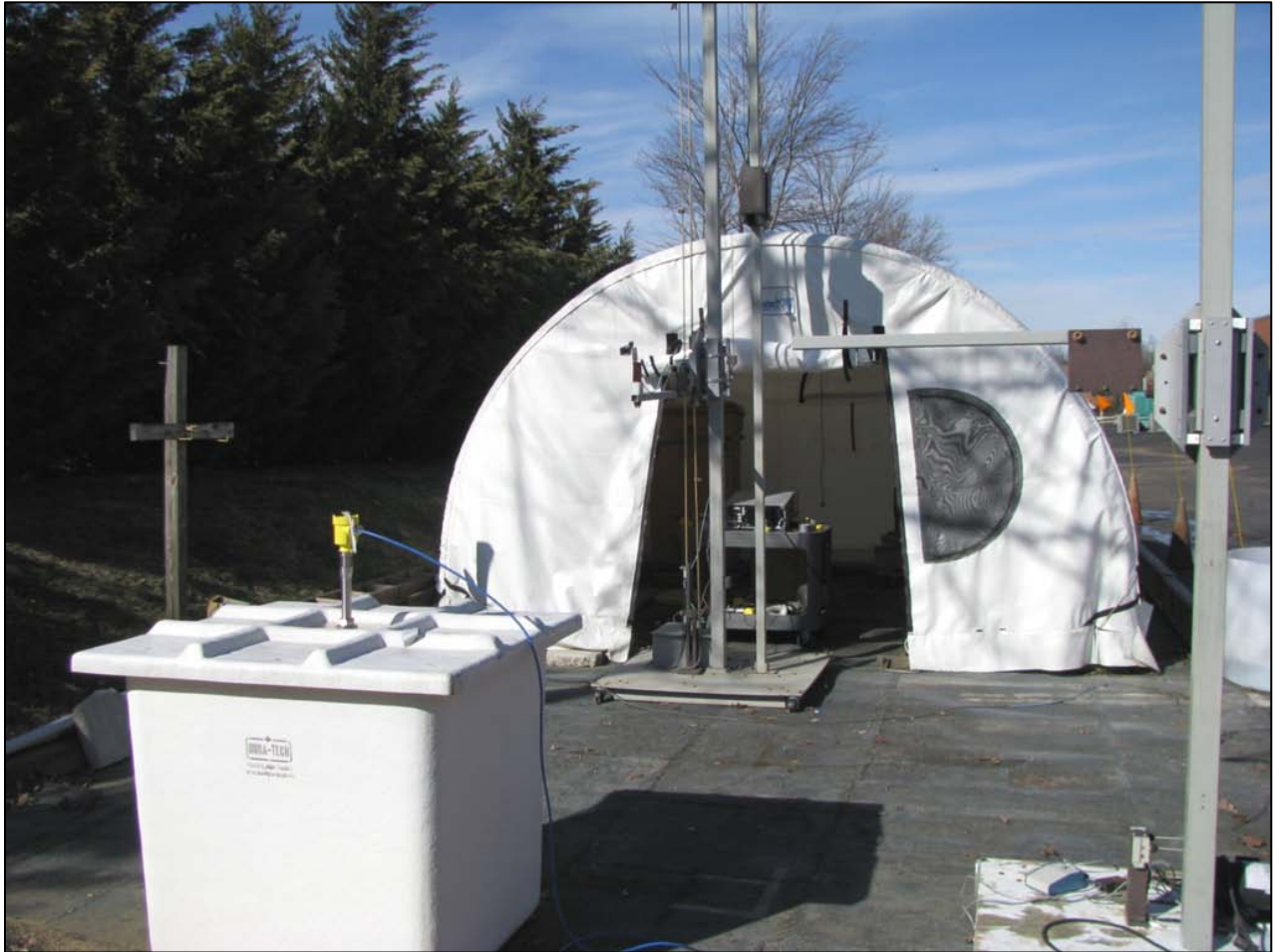
Photograph 38: 95mm Antenna Rear View Fiberglass Tank
