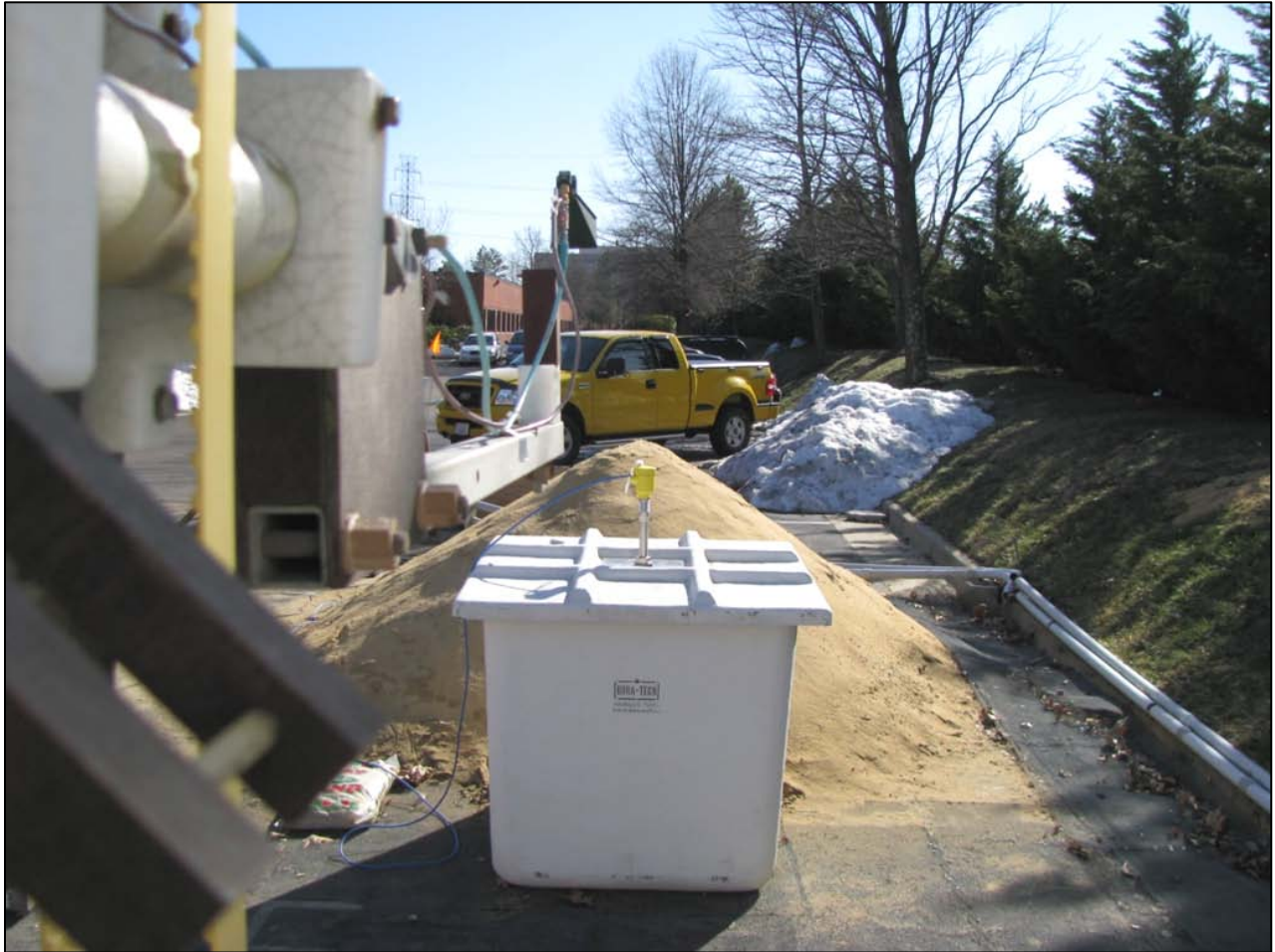
Photograph 37: 95mm Antenna Front View Fiberglass Tank
