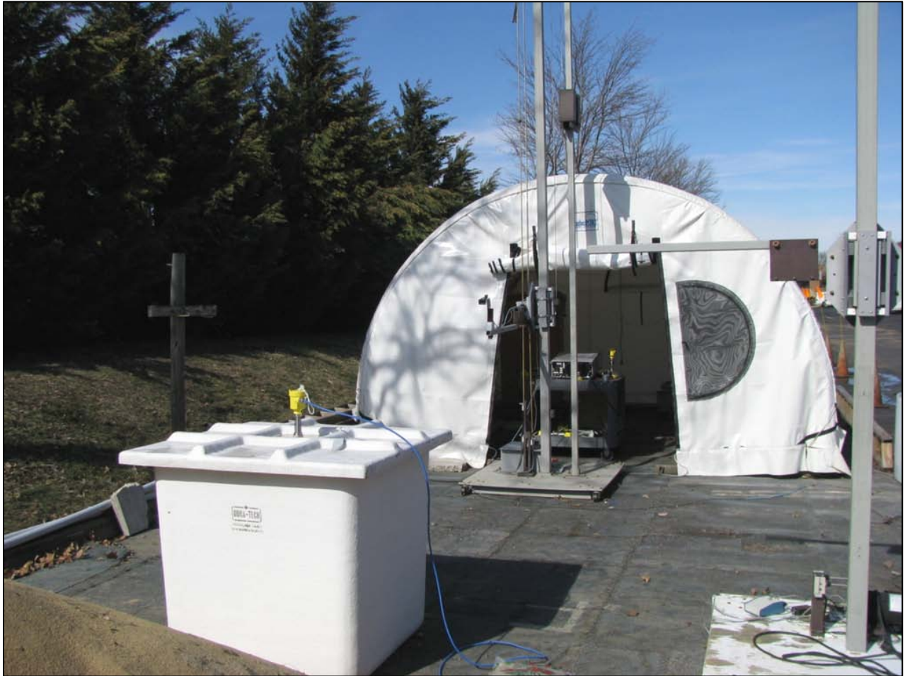
Photograph 36: 245mm Antenna Rear View Fiberglass Tank
