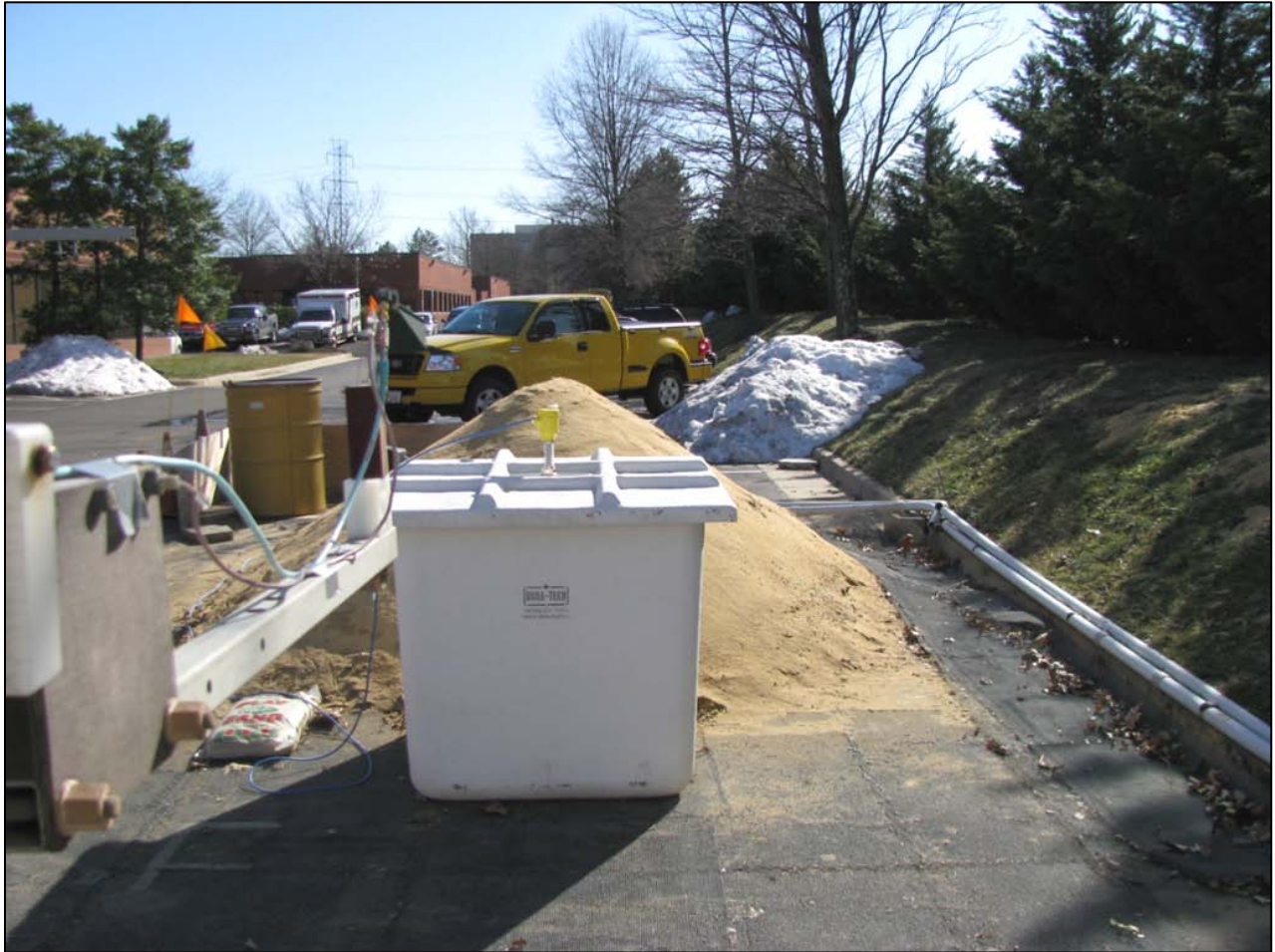
Photograph 49: ½” Standpipe Antenna Front View Fiberglass Tank
