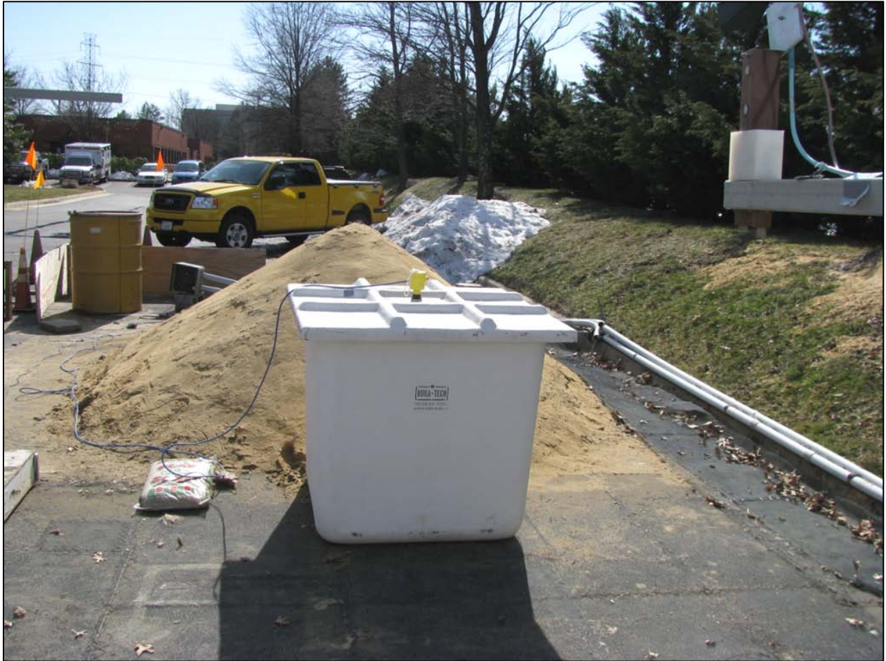
Photograph 47: 1/2" Stub Antenna Front View Fiberglass Tank
