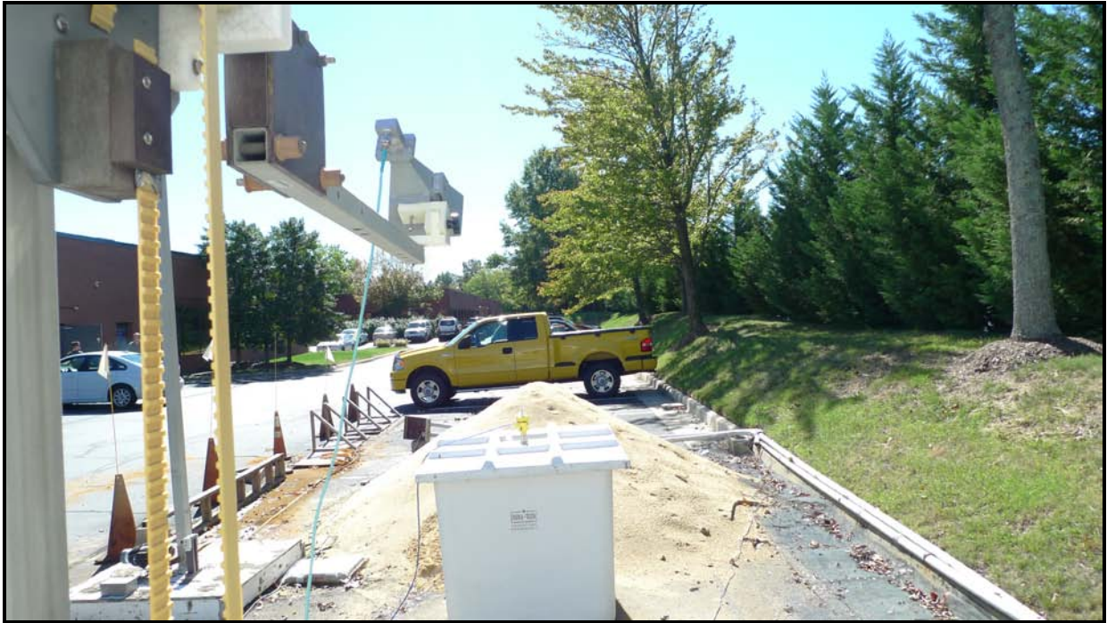
Photograph 19: 10" Horn Antenna Front View Fiberglass Tank
