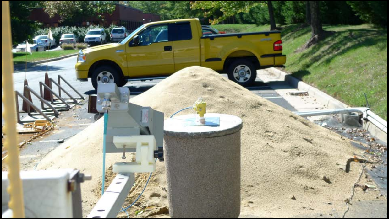
Photograph 17: 50mm Rod Antenna Front View Concrete Tank
