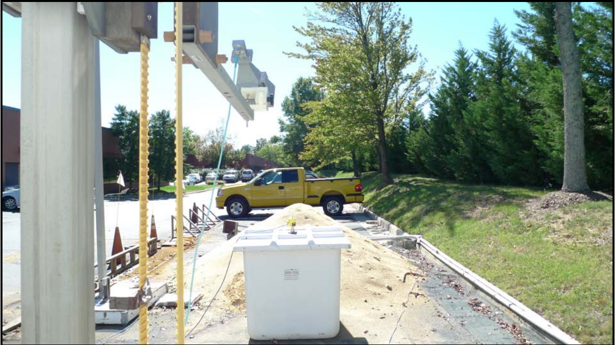
Photograph 21: 4" Horn Antenna Front View Fiberglass Tank
