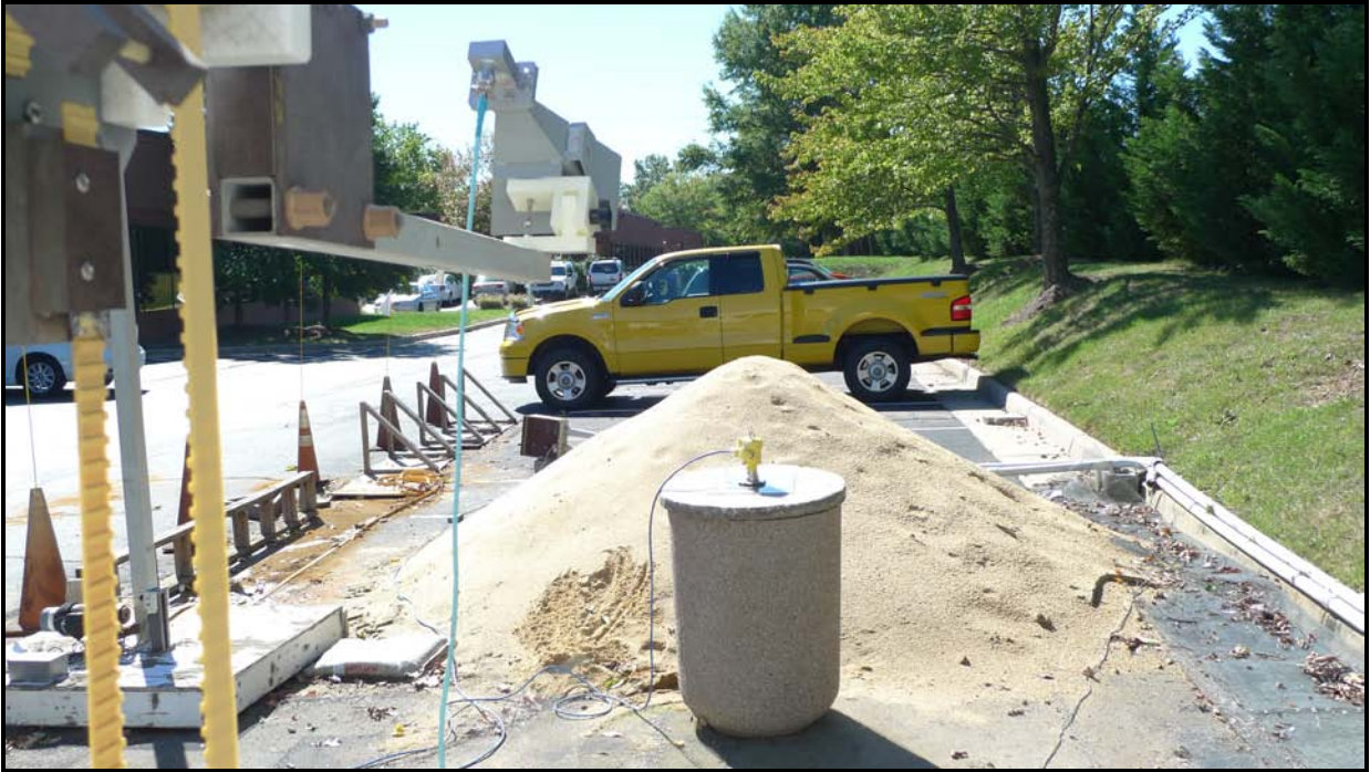
Photograph 15: 250mm Rod Antenna Front View Concrete Tank
