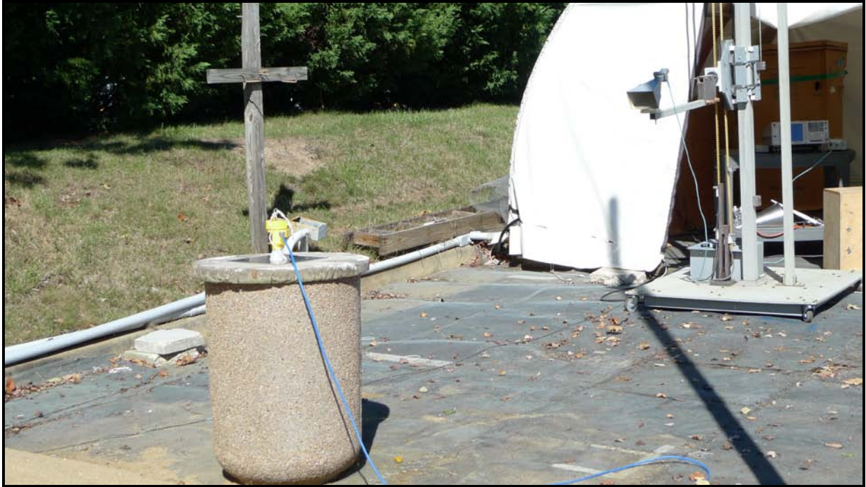
Photograph 18: 50mm Rod Antenna Rear View Concrete Tank
