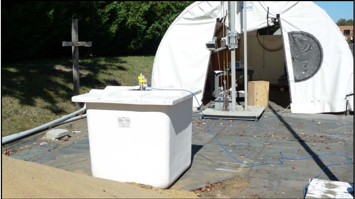
Photograph 20: 10" Rod Antenna Rear View Fiberglass Tank
