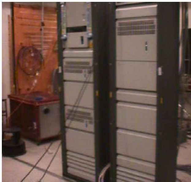
Photograph of Antenna Conducted Spurious Emissions Test Configuration
