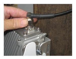
Figure 33 – Connecting the antenna RF cables
