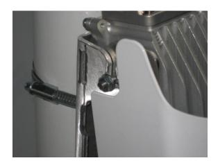
Figure 26 – AirSynergy drops down into slots at the top of pole-mount plate
