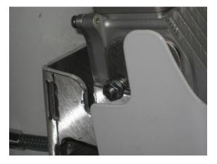
Figure 25 – Lift AirSynergy to top of pole-mount plate
