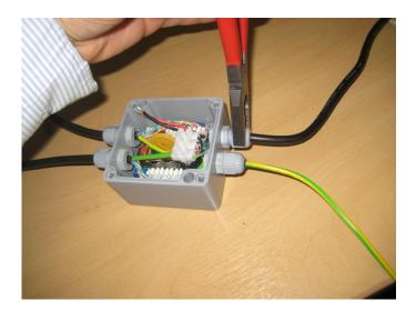
Figure 50 – Pass the d.c. power cable through the gland and tighten the end cap
