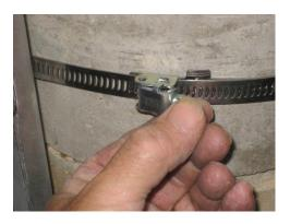
Figure 17 - Press down the locking mechanism with the slack band fed through
