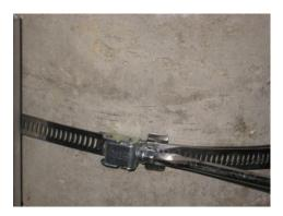
Figure 18 – Tighten clamps with large flat blade screwdriver
