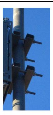
Figure 65 - Mounting method with pole clamps recommended for back to back installations
