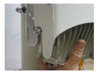
Figure 27 – Gently lift the AirSynergy body until the bottom studs engage in the bottom slots
