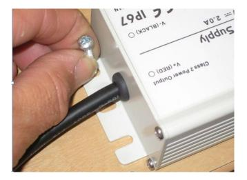
Figure 54 - Fix the PSU into position using self tapping screws
