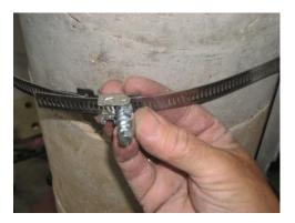
Figure 16 - Feed clamp bands through the quick release locking mechanisms
