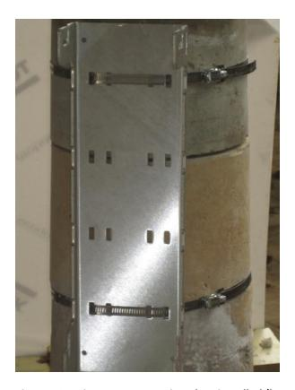
Figure 19 – AirSynergy mounting plate installed (large diameter concrete pole)
