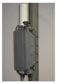
Figure 67 - Back to Back AirSynergy mounted on pole with 4 mounting straps
