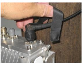
Figure 34 – AirSynergy Front mount antenna connections – applying self -amalgamating tape
