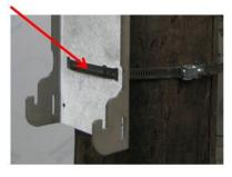
Figure 66 - Flatten straps against the mounting plate for back to back installations
