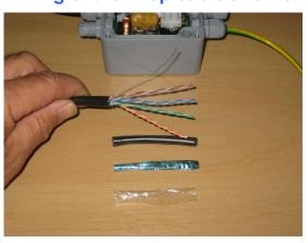
Figure 39 – Preparing the drop cable/network cable wire ends for connection into the PoE injector
