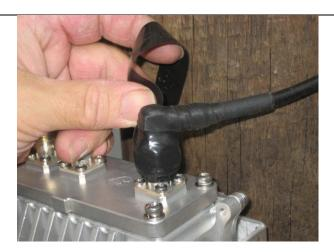
Figure 35 – AirSynergy antenna connections – applying PVC tape Ensure the RF connector is completely sealed from the weather.
