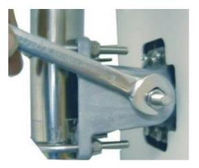
Figure 19 - HiperMAX-micro SCRT attach SCRT and antenna to pole
