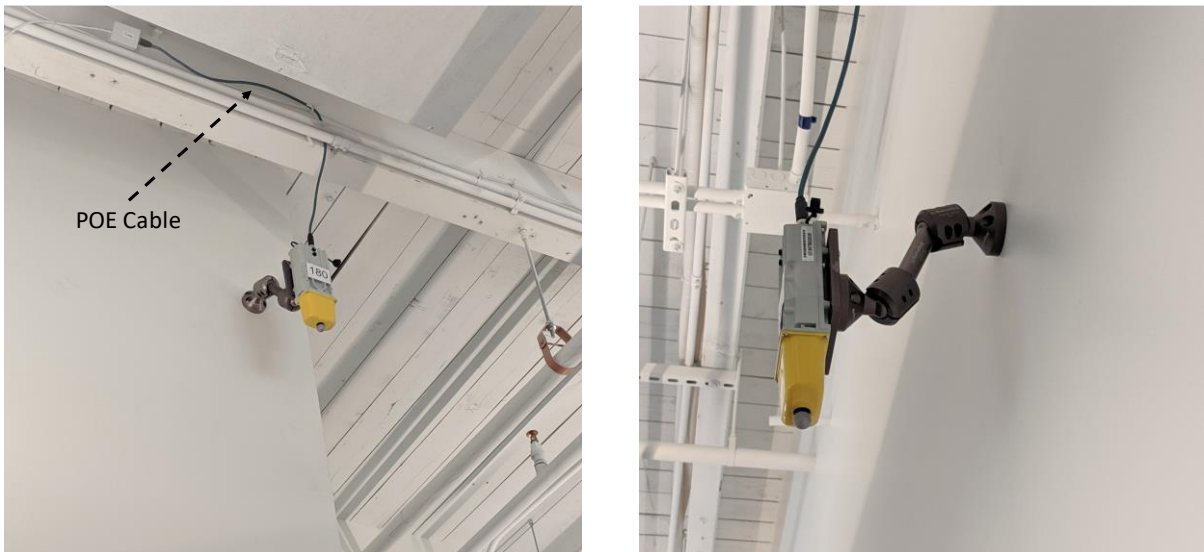
Fig. 6: Example inbuilding wall mount using standard VESA mounts. Routing of the POE cable is also shown.
