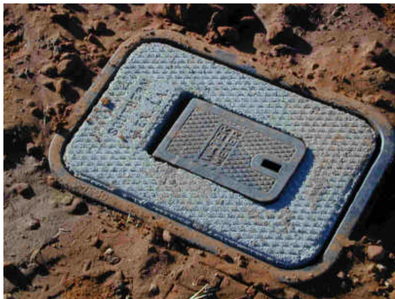
Photograph 3.2.4 Plastic pit Concrete cover with metal lid
