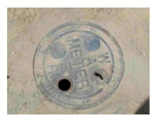
The metal pit must be completely buried in the ground with its cover at ground level as shown above.
