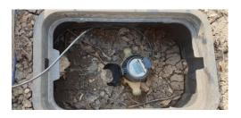
**Step 2)**Remove threaded locking mechanism
