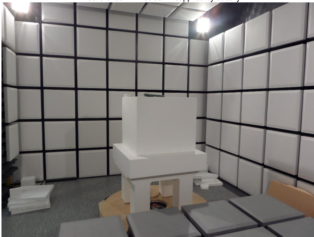
Anechoic room – Position 2 supplied by battery
