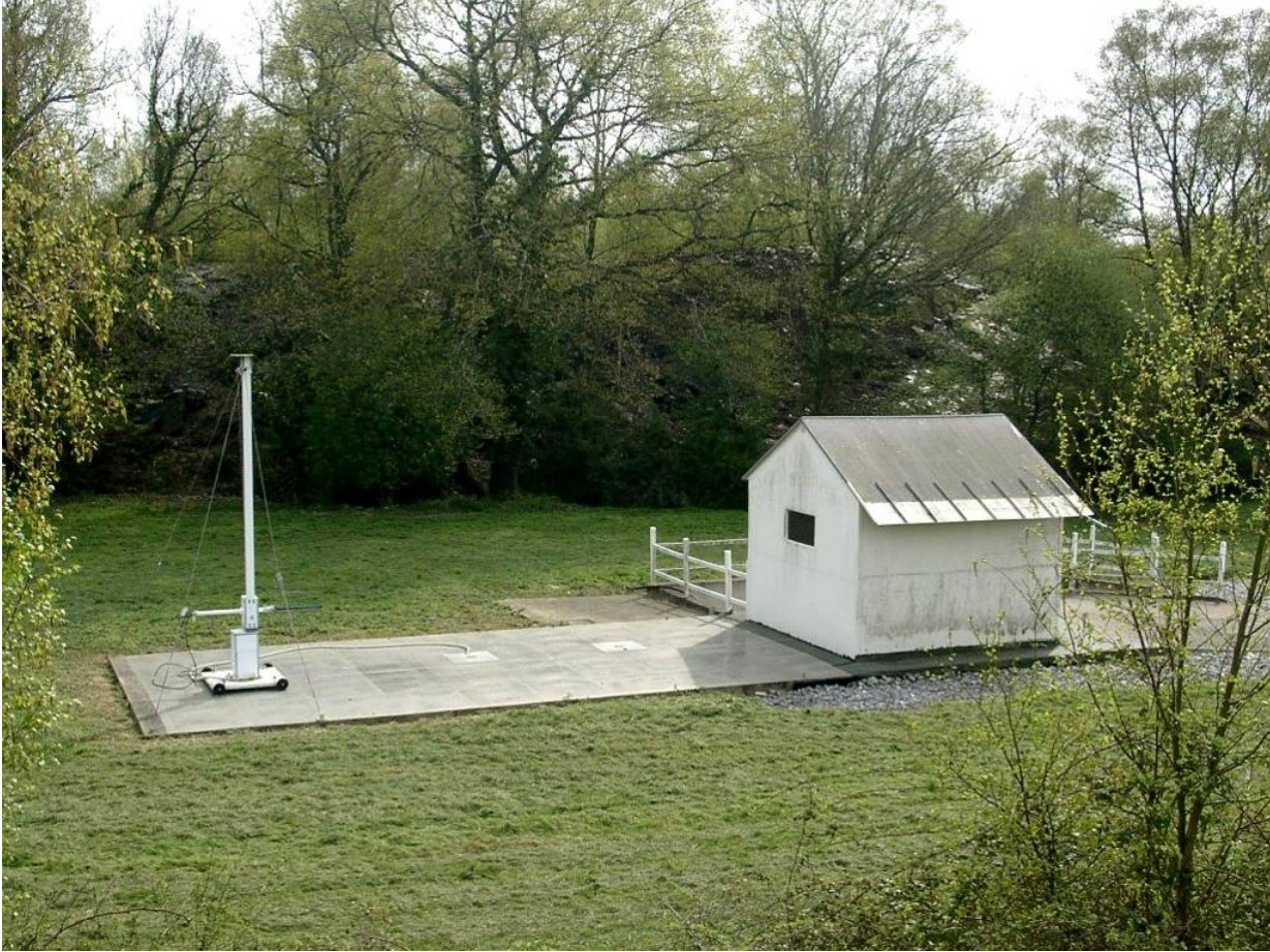
Open Area Test Site (test antenna at 10m)
