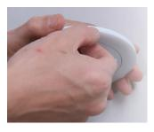
Step 3. Place the bracket on the wall and mark the pilot hole locations.
