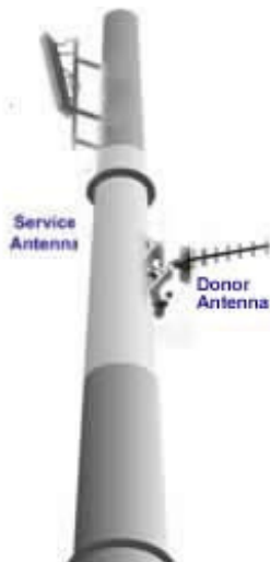
Figure 2-1. Service above Donor Antenna
