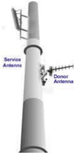
Figure 2-1. Service above Donor Antenna
