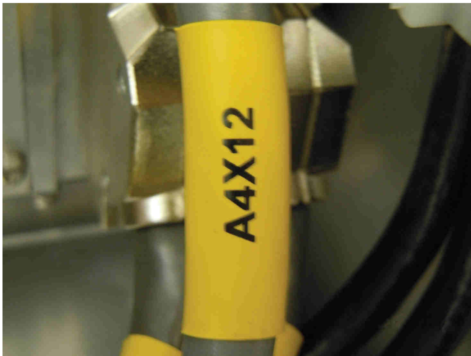
Fig. 10.5 Marking, other cables
