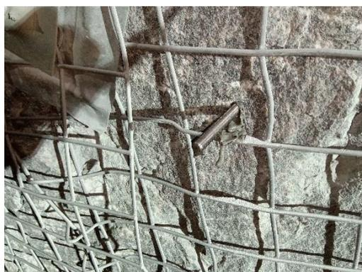
Plate Step 3. Insert both Anchors
