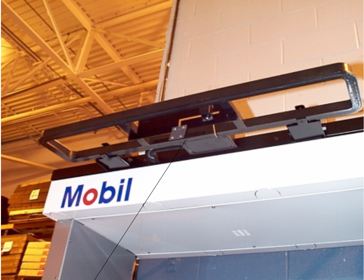
View showing overhead antenna for car mounted tag application
