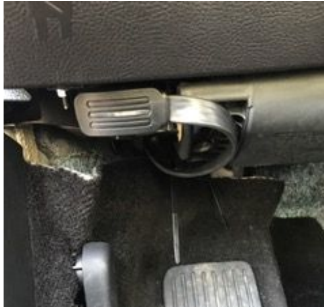
UTP 1.0 installed on 2017 Ford Fusion. UTP is routed and tie wrapped onto a wire harness behind the panel.
