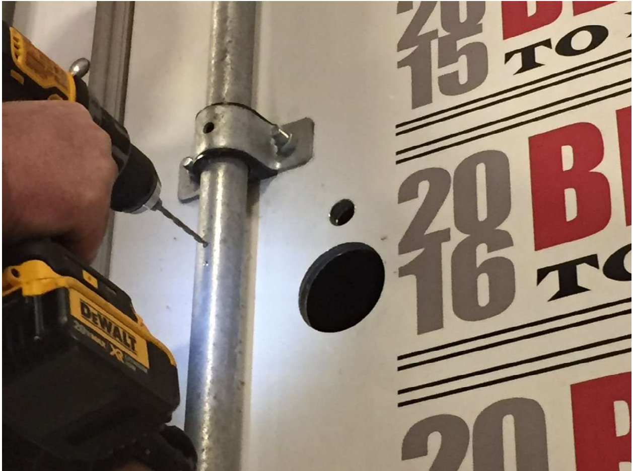
Drill #17 holes in inner locking rod
