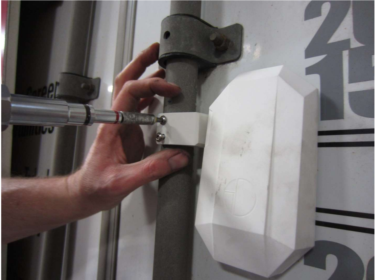
Install thread forming screws
