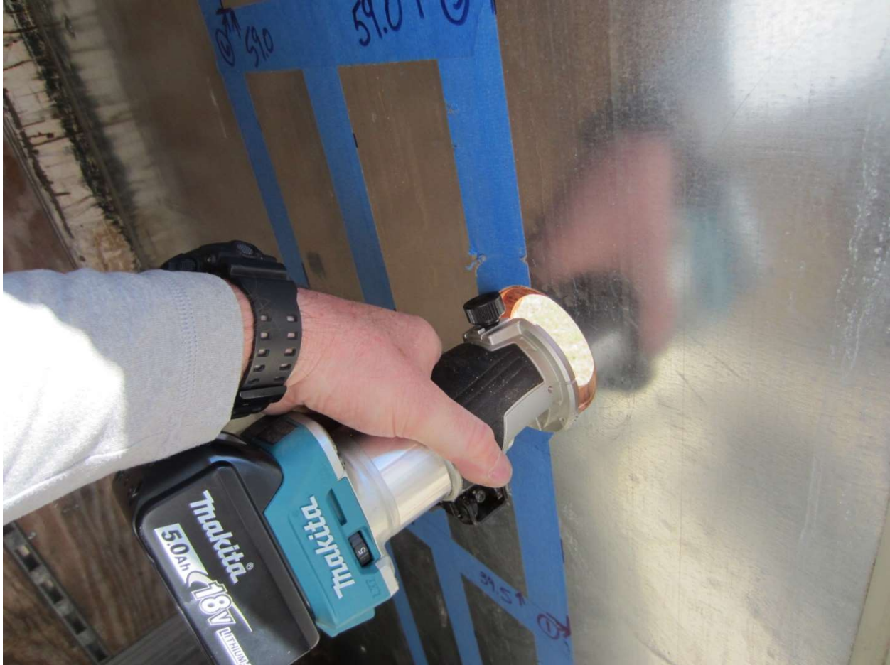
Create countersink with router
