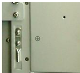
Figure 4-2 Ground Cable Connection
