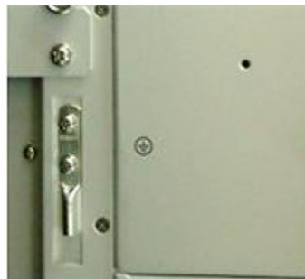
Figure 4-2 Ground Cable Connection
