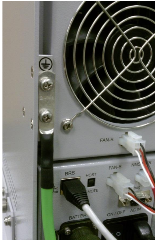
Figure 22 Ground Cable Connection
