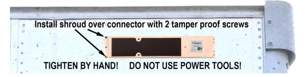
Fasten the Short Shroud to the SkyHub with two, 10-32 tamper proof screws
