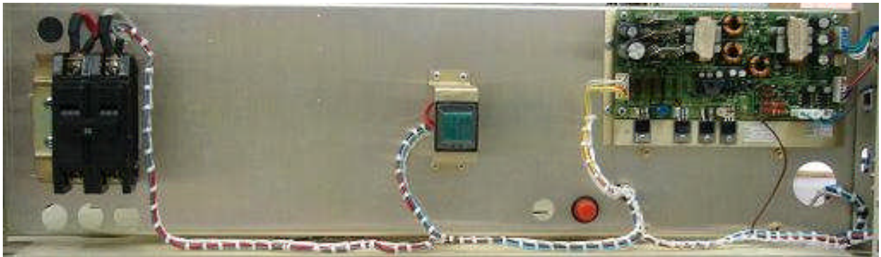
Fig.7.1: Energy Distribution – Bipolar Main Breaker on left, manual starter on the center and module 4147 – battery charger.
