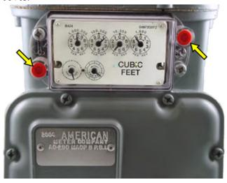
1. Remove the four screws from the clear index cover.
