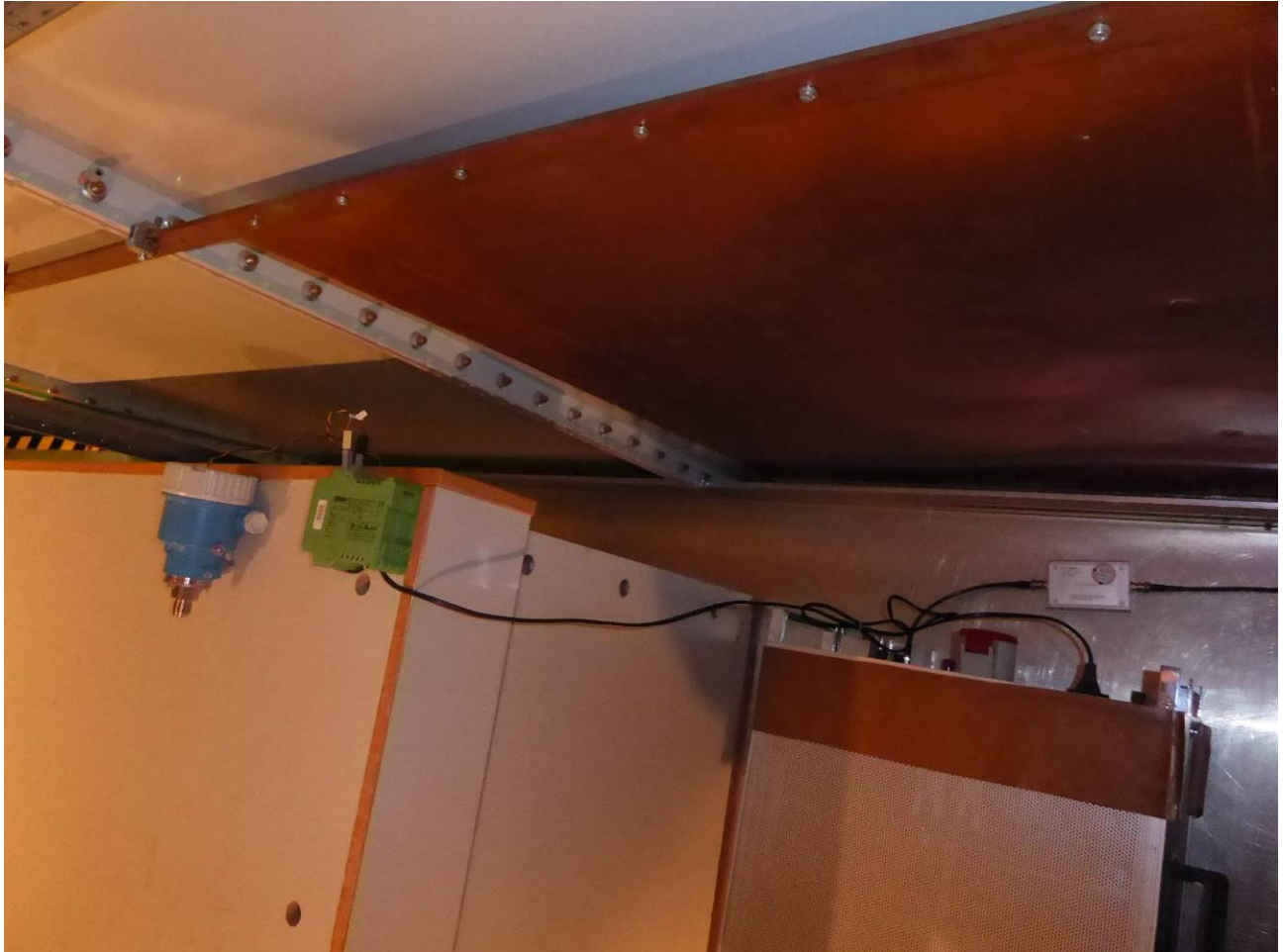
Test setup – conducted emissions on power supply lines
