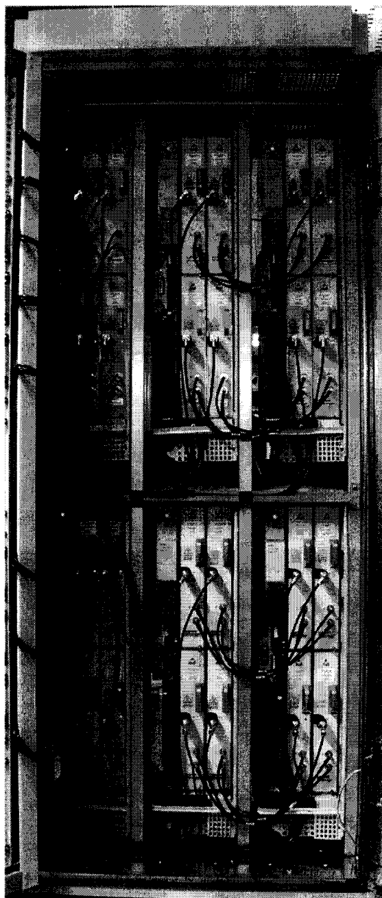
Figure 12. HcHc cabinet shown with units fitted
