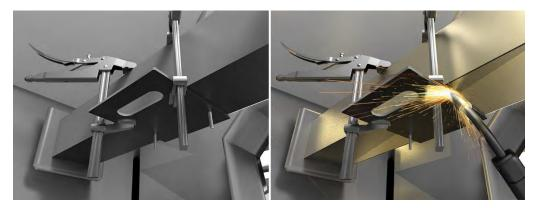
**IMPORTANT:** If you are welding the bracket to your asset; it is recommended to remove the Radar R2 IS module from the bracket before welding the bracket to the rail car. While the Radar R2 IS module can be mounted to the bracket, before the bracket is welded to the railcar, it is the responsibility of the installer to ensure the Radar R2 IS module is protected from weld splatter and extreme temperatures.
