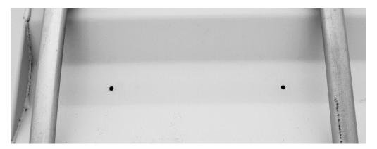
2. Insert the nuts and bolts into the holes. For added protection, place a washer between the bolt and the door surface.
