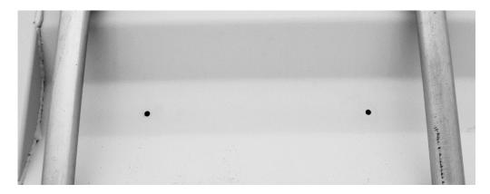
2. Source a set of nylon or rubber plugs, of the appropriate diameter, to fill the holes. These plugs can be sourced from hardware or auto supply stores. Insert the plugs into the holes. If desired, you may add 100% Silicone Exterior Grade caulk to the rear of the plug for extra protection to seal any gaps against water entry.
