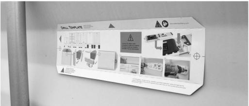
3. Using a drill bit, drill a hole through each of the cross hairs on the template. This will create two holes you will use to mount the module.
