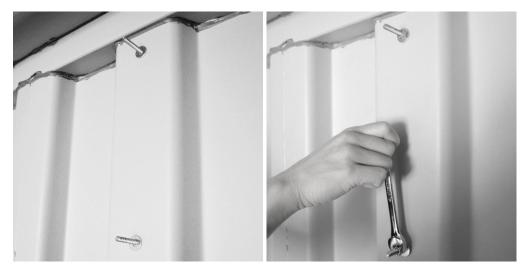
**Tip:** If, when installing the nut on the carriage bolt, the carriage bolt becomes dislodged from the module, you may complete the installation of the nut by grasping the threads of the bolt with a set of pliers, pulling the bolt to reset the square neck into the pocket and tightening the nut with a wrench.
