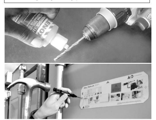
4. Remove the template. You now have two holes in the door. If there are any burrs around the holes, remove them at this time. Also, remove any dust or debris left over from the drilling or de-burring operations and ensure surface is clean and dry.
