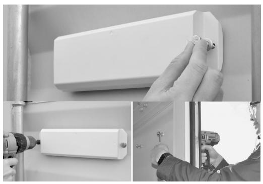
Do not over-tighten the fastener. Over-tightening can over-compress the mounting pad, which can damage the pad. Do not tighten fastener beyond 35 in-lb. (4N-m).
