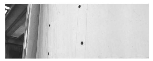
2. Fill the holes with a weatherproof sealant. If desired, you may use 100% Silicone Exterior Grade caulk or Polyurethane Sealant.
