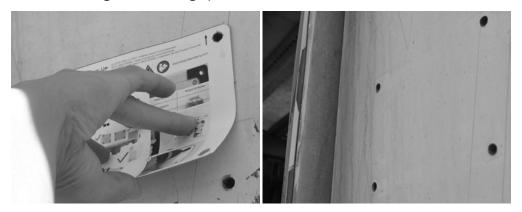
6. Place the module on the door, aligning the holes on the module with the holes you drilled into the door.
