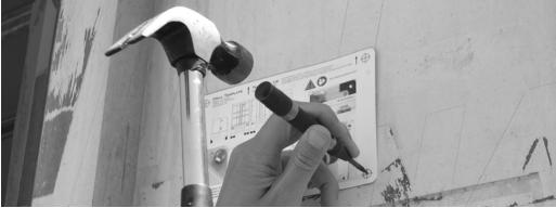
5. Remove the template. You now have four holes in the door. If there are any burrs around the holes, remove them at this time. Also, remove any dust or debris left over from the drilling or de-burring operations.
