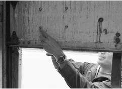
**IMPORTANT:** If you are using the lower door placement location, it is important to completely raise the door through its full range of travel, then lower the door completely, to initialize the door orientation sensor. Performing this operation allows the door to learn the difference between a door open and door close event.
