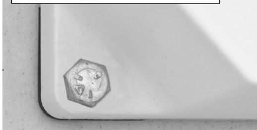
Gasket Compression Level Recommended
