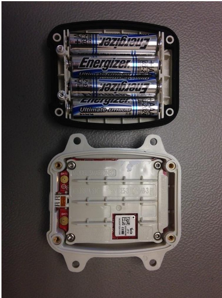
S1C Opened with batteries installed
